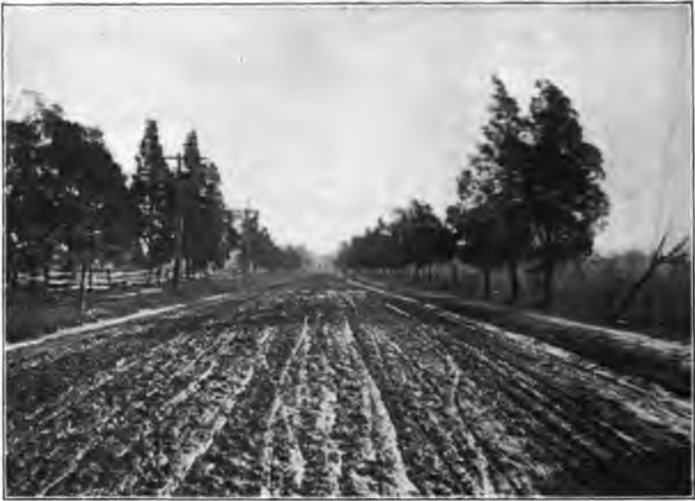
New Brunswick and Bound Brook road, Middlesex Co., before improvement.
